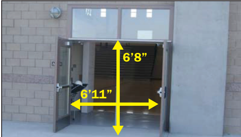
PERF. ENTRANCE “OUTSIDE VIEW”
