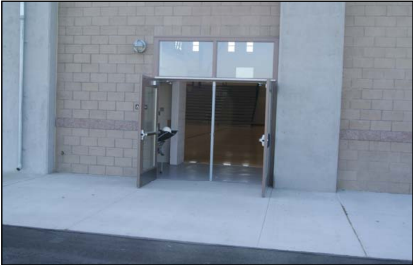
PERF. ENTRANCE "OUTSIDE VIEW"
