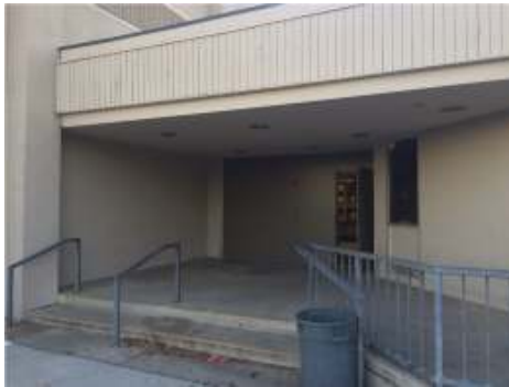
Performance Entrance Area (outside view)
